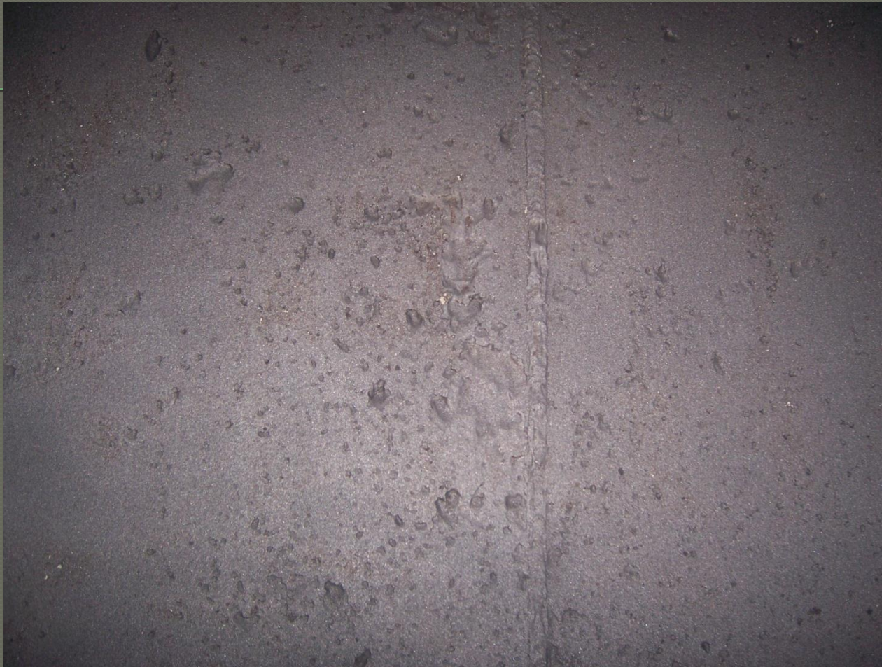
Inside Tank, Vertical Weld
